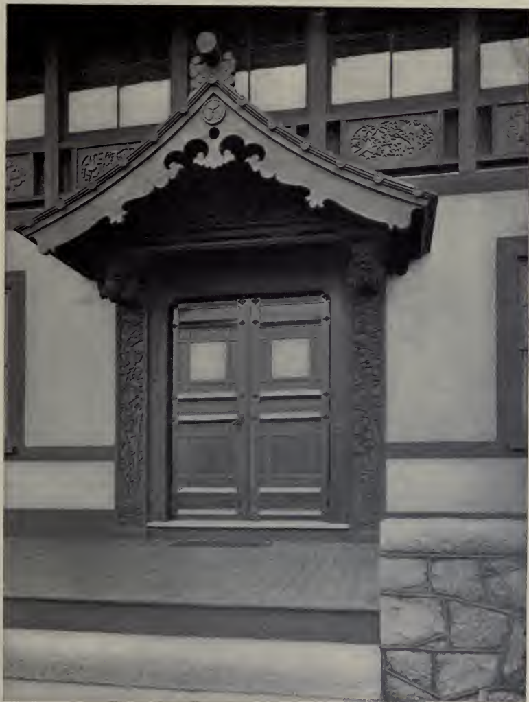
DETAIL OF THE FRONT DOOR.
