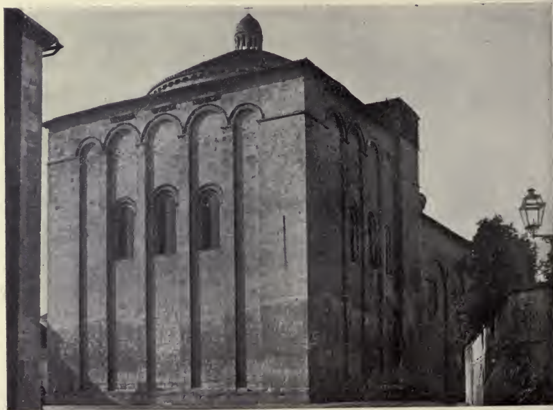
S. ÉTIENNE, PÉRIGUEUX. (From the northeast.)
