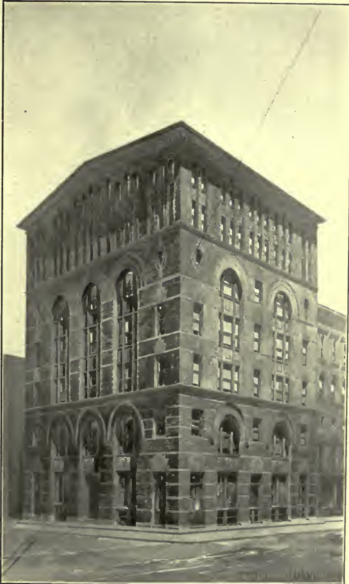
FIG. 7.—THE TARRANT BUILDING.
