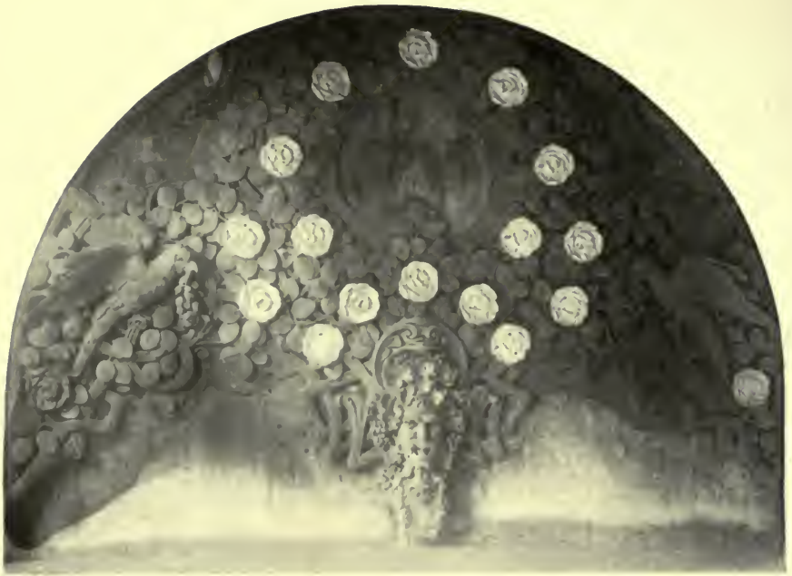
DETAIL IN THE NEW AMSTERDAM THEATRE.
