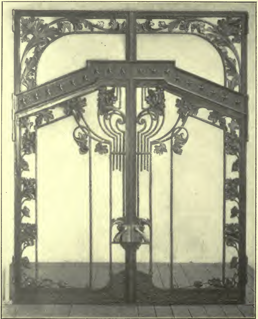
IRONWORK, NEW AMSTERDAM THEATRE.
