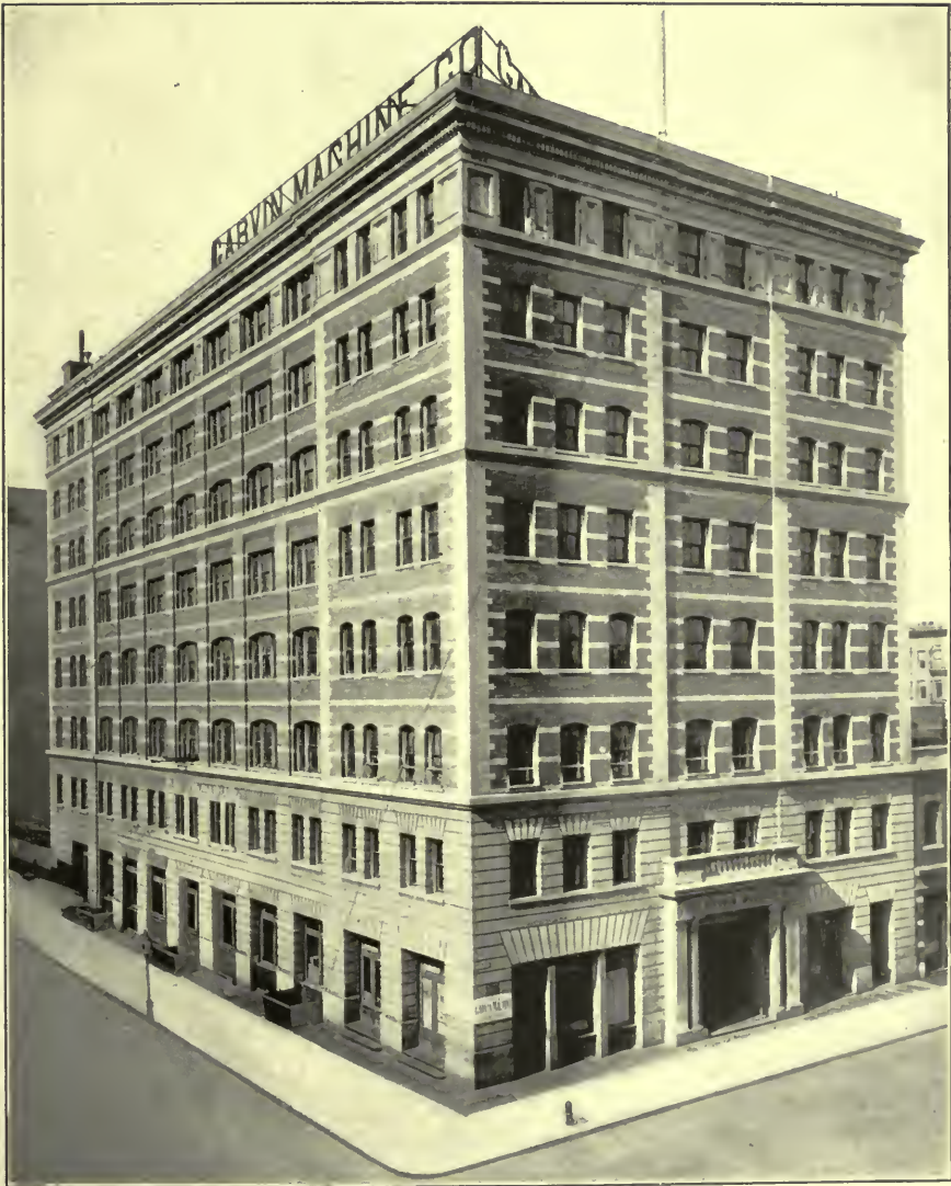
FIG. 8.—BUILDING OF THE GARVIN MACHINE CO.
