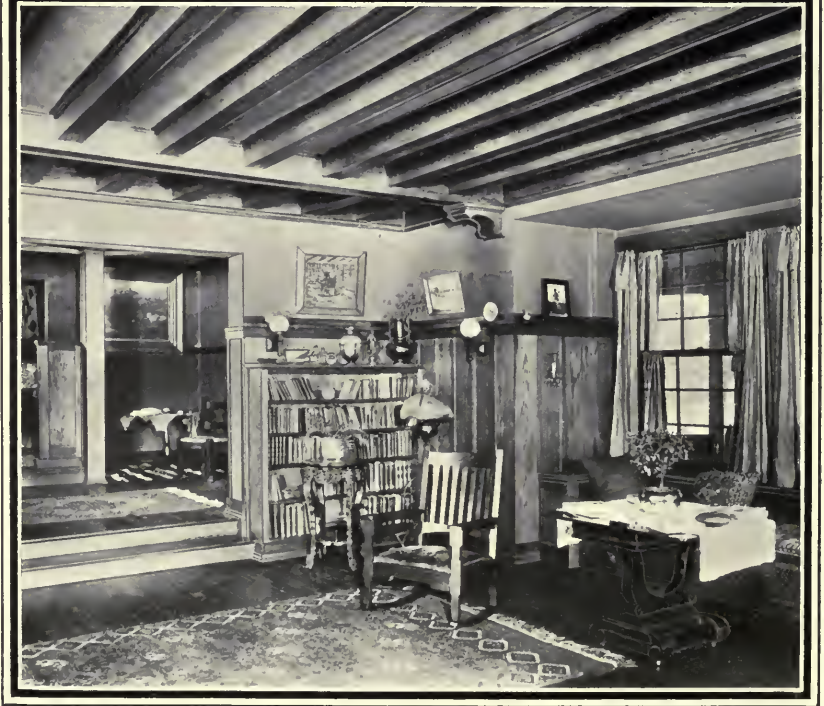
FIG. 11.—HALL IN THE HEALY HOUSE. Chicago, Ill. Myron Hunt, Architect.
