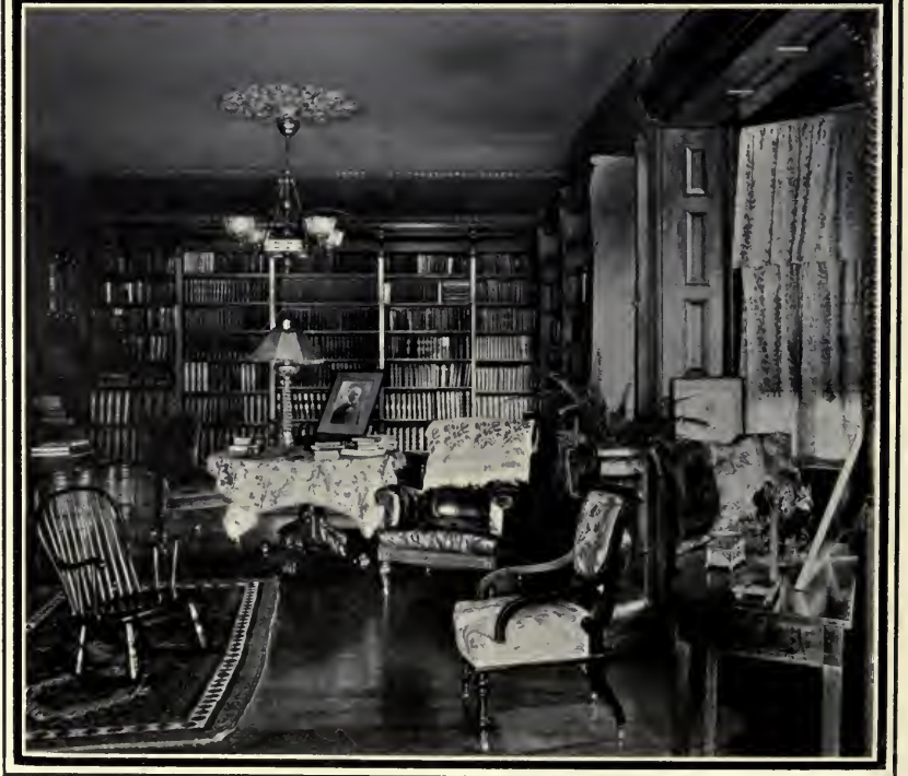
FIG. 40.—LIBRARY IN THE WILCOX HOUSE. Buffalo, N. Y. Geo. Cary, Architect.
